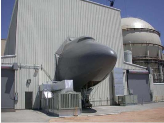
The System Integration Lab (SIL) at Edwards AFB, Calif., where the tests on the Chemical Oxygen Iodine Laser (COIL) were conducted in the interior of the Boeing 747 fuselage, whose nose is protruding through the metal wall. USAF Photo.
