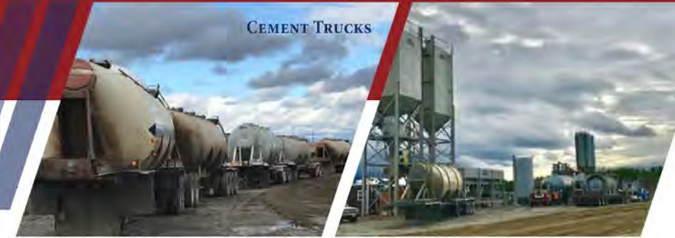
4,100 cubic yards (cy) of cement was placed in 19 hours for the radar foundation at CSFS, which is the second largest continuous concrete pour in the state of Alaska, averaging approximately 243 cy/hr.
