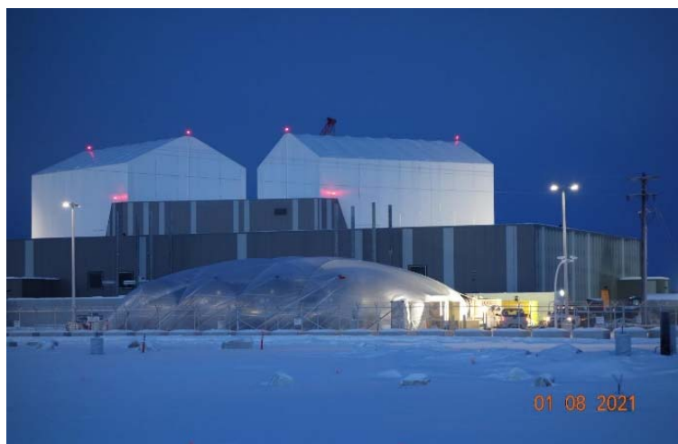
Rear view of LRDR, Clear AFS. The white structures are Array Assembly Areas used only for Environmental Protection during radar installation.
